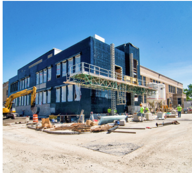
Construction of George Mather Forbes School 4
